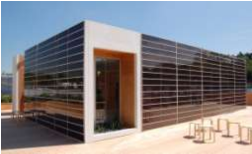
PV Ventilated Façade for the SML House, Solar Decathlon Madrid
