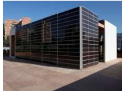
PV Ventilated Façade for the SML House, Solar Decathlon Madrid
