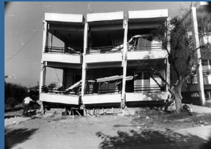
Fig. 27 Ground problems accompanied by heavy structural damage in R/C columns (RED)
